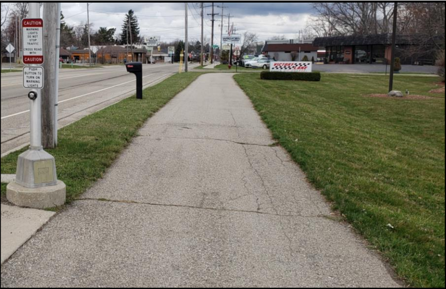
Location F: Transverse Cracking
