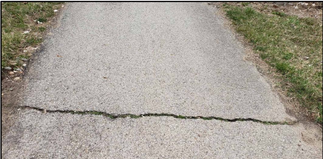
Location A: Transverse Cracking
