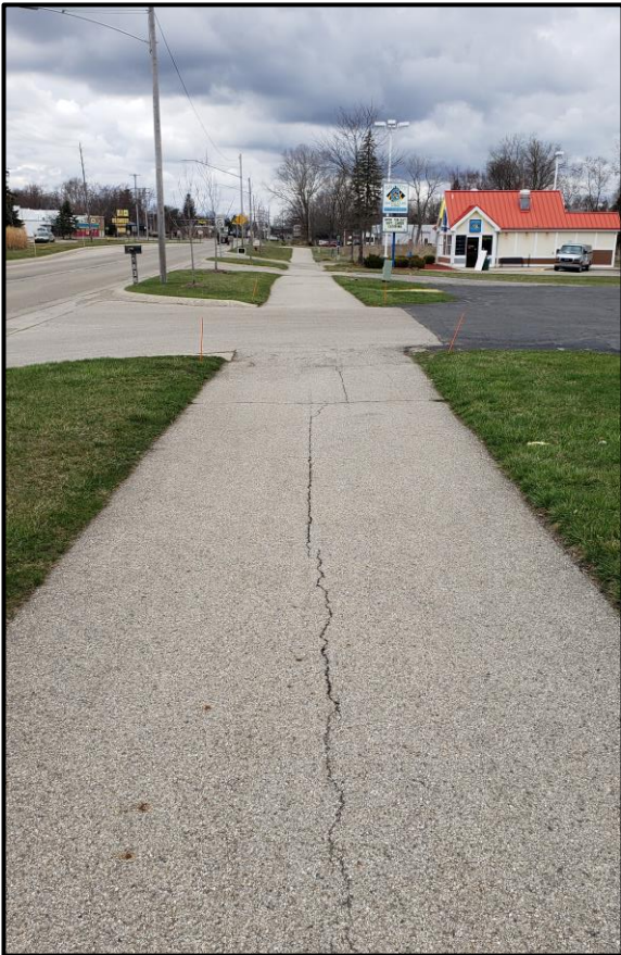
Location D: Longitudinal & Transverse Cracking
