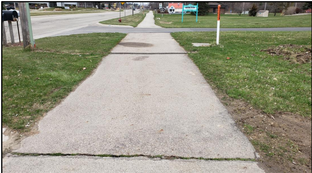
Location C: Transverse Cracking
