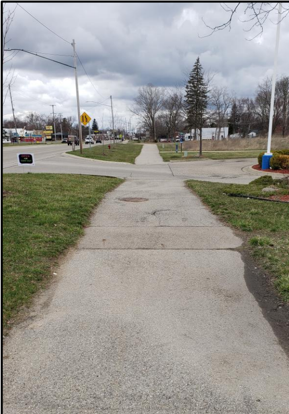
Location E: Upheaval & General Disrepair (Full Depth Replacement)
